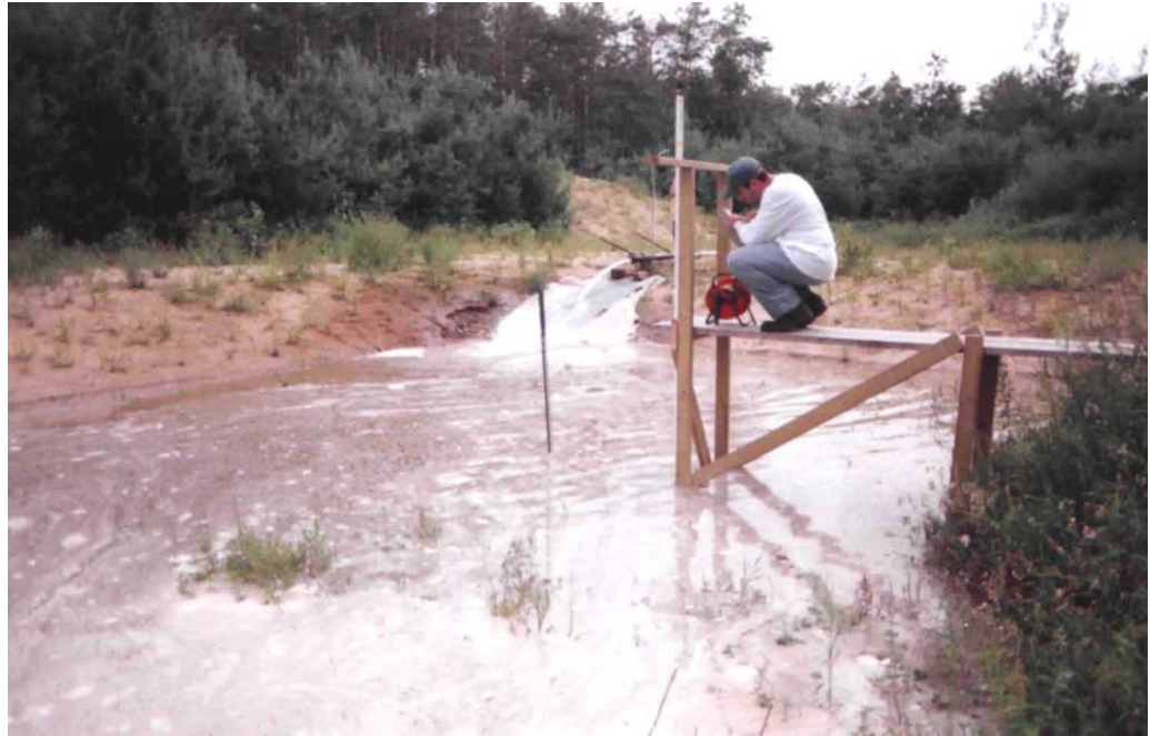
Figure 4: Lagoon with sand embankment on HDPE geotextile liner
