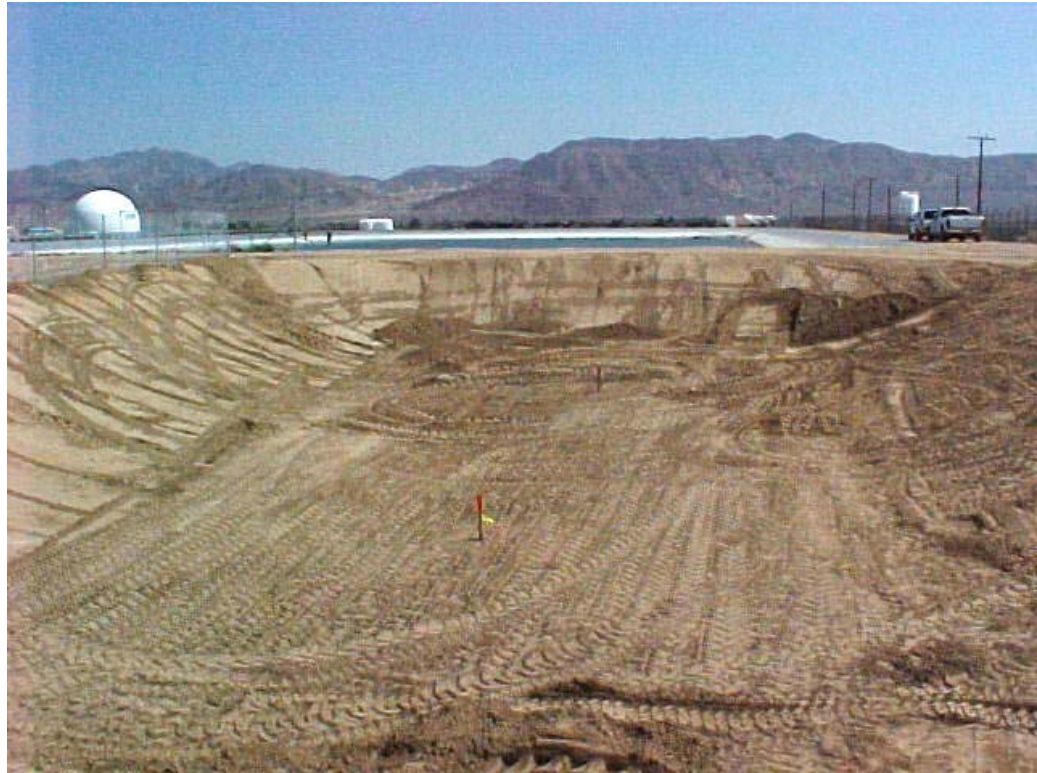
Figure 2: Lagoon excavation
