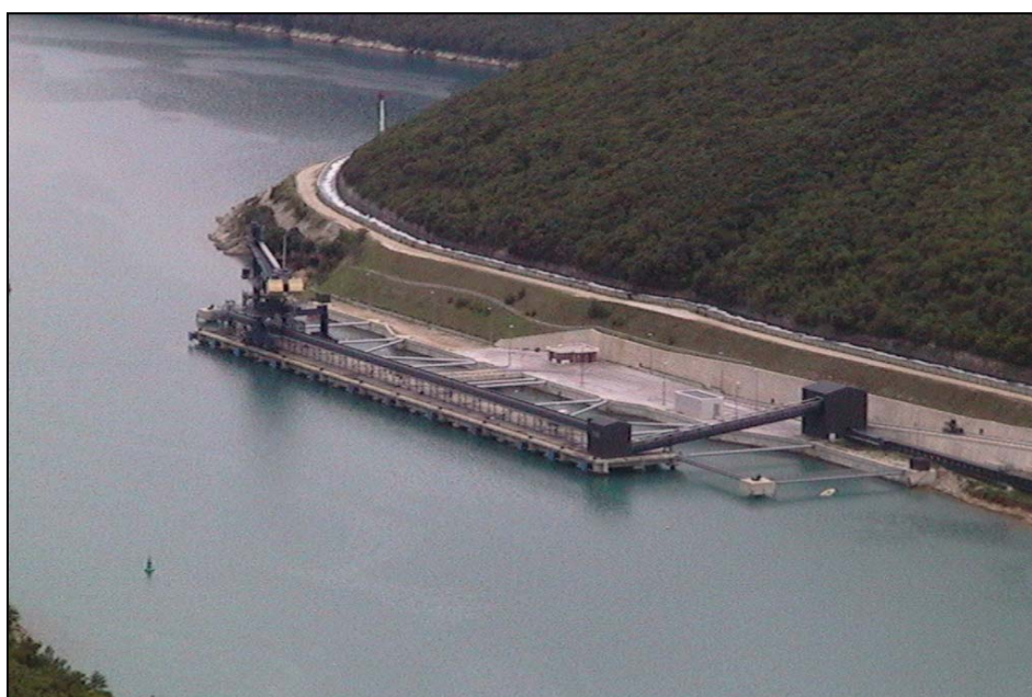
The discharging wharf of the terminal
