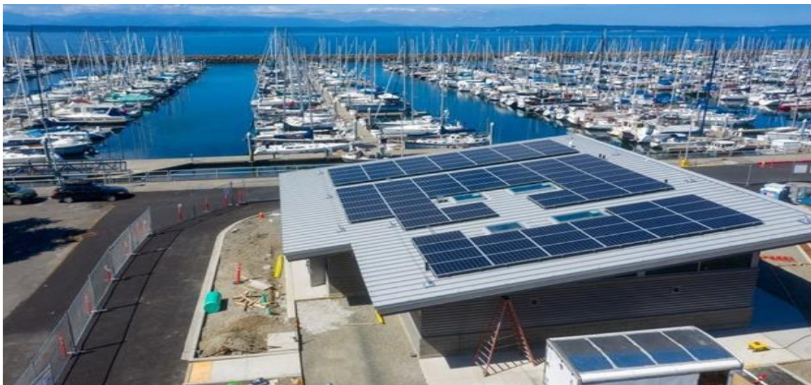
Figure 5.22 Solar power generation in a port
