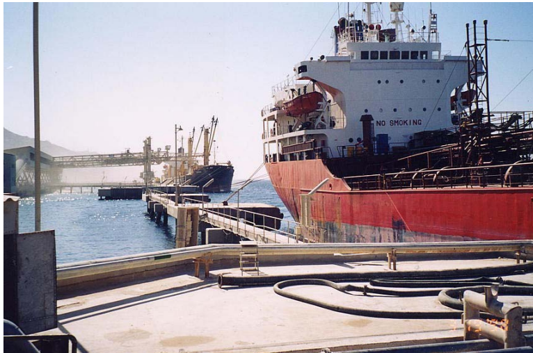
Photo.1 View of the terminals in the Main Port
