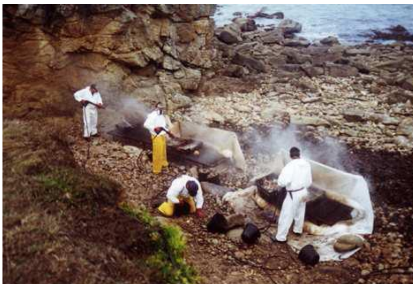
Washing of pebbles on site (Source: Cedre)
