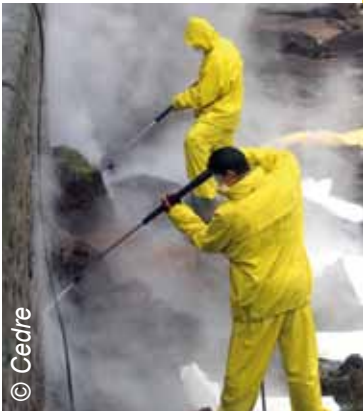
Booms and sheets deployed to trap thermal washing effluents
